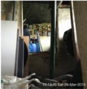
Unsafe Score Box Area
